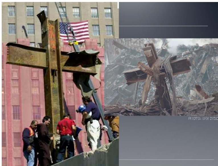
The cross of steel. Many of the remaining columns and beams looked like crosses rising from the smoke and ash that was ever present for months.
